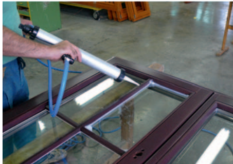
glazing windows with silicone
