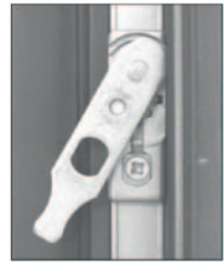
catch securing the handle against turning
