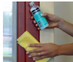
removing impurities using the supplied cleansing agent
