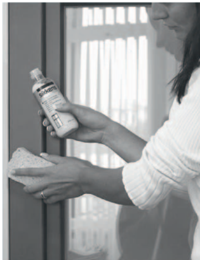
surface treatment using supplied milk
